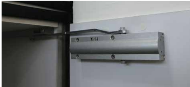
When the temperature reaches 50 °C, the doors close automatically.
